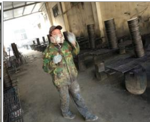
Photo of non-conformity Employees did not properly wear PPE (Personal Protective Equipment).jpg
